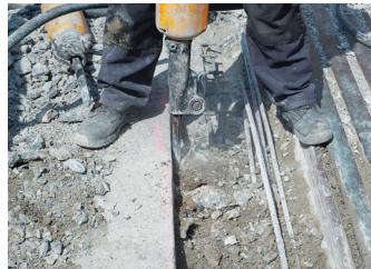
Pavement Removal
