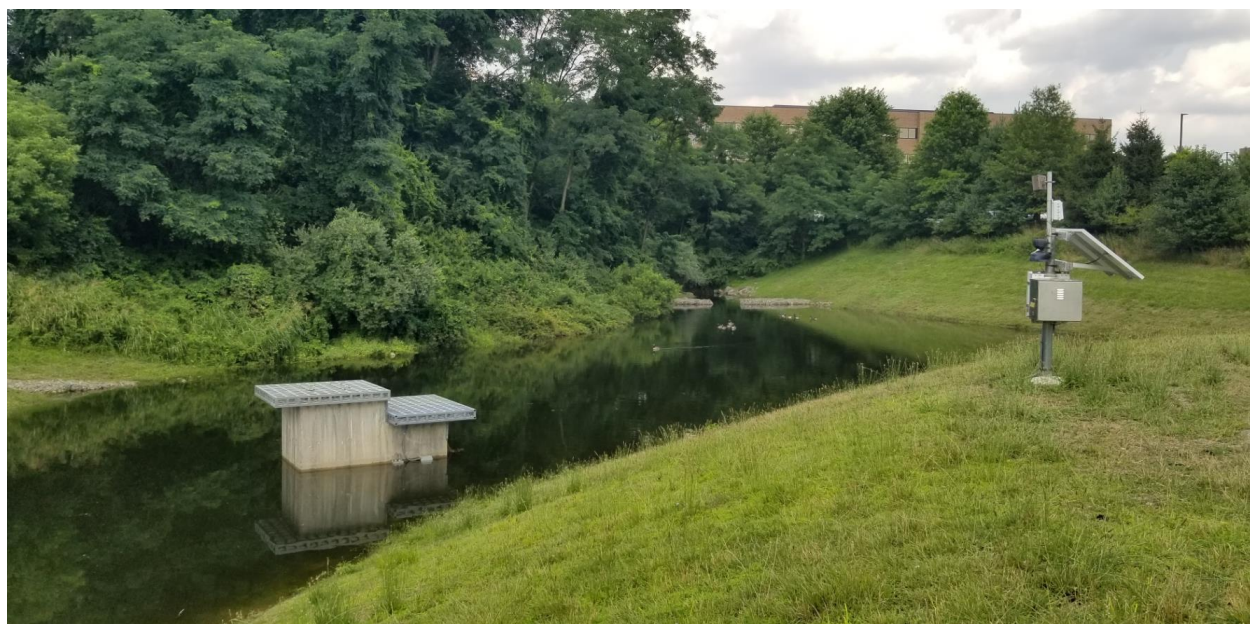
Image: WalMart pond after 2018 retrofit
