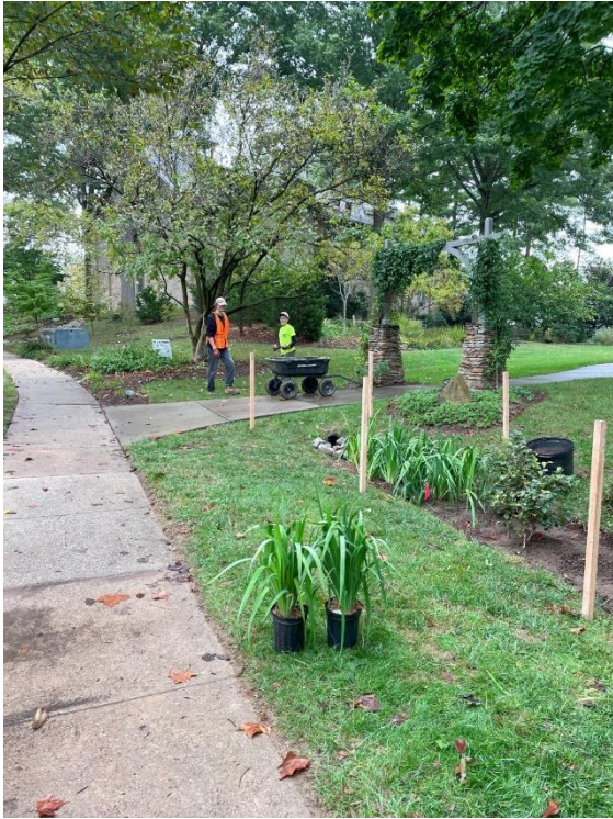
Bioswale installed at Kittamanqundi Community Church
