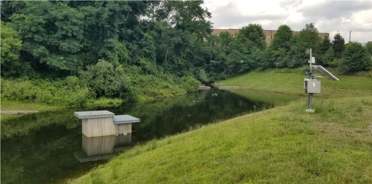
Image: WalMart pond after 2018 retrofit
