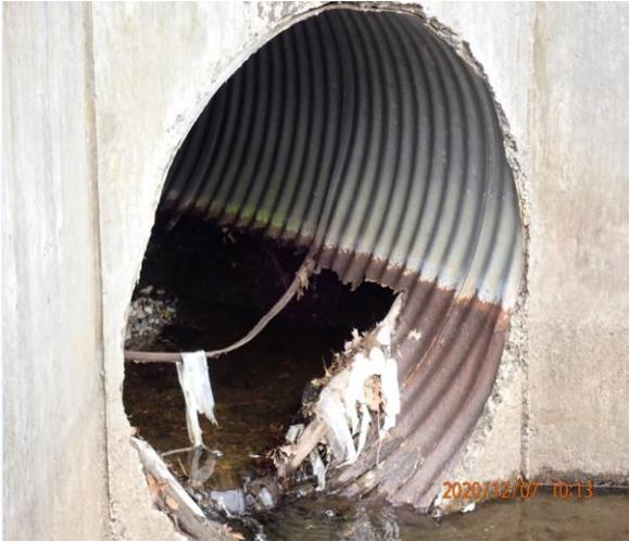
Stormwater culvert with significant damage to bottom and sides, allowing erosion of surrounding soil and compromising the structural integrity of the system, which will lead to road collapse.
