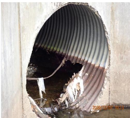
Stormwater culvert with significant damage to bottom and sides, allowing erosion of surrounding soil and compromising the structural integrity of the system, which will lead to road collapse.
